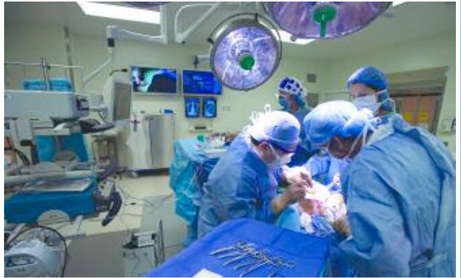
Ceiling-mounted booms help keep cords off the floor and improve ergonomics.
